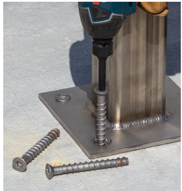
Titen HD Countersunk Installation
