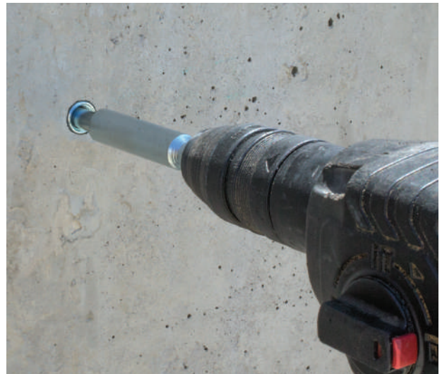
Anchor being set with SDS setting tool.
