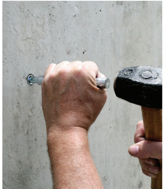
Anchor being set with hand setting tool.
