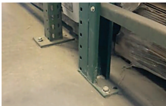
Typical low-corrosive environment — interior warehouse.
