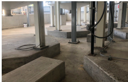
Typical medium-corrosive environment — exterior anchorage.
