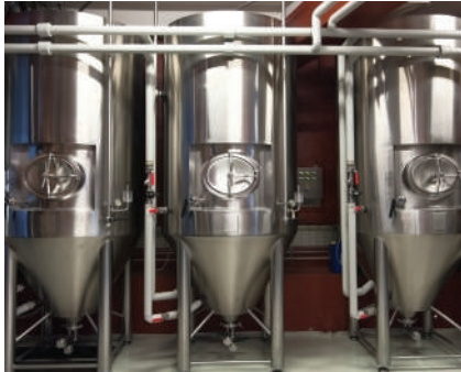
Typical high-corrosive environment — food-processing plants.
