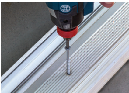
Sliding door track installation
