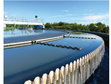
Typical severe-corrosive environment — wastewater treatment plants.
