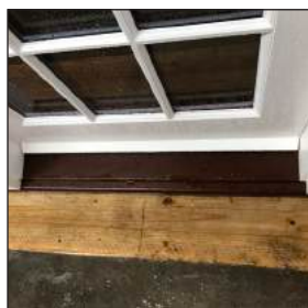
Stepped wooden sill crafted out of multiple pieces
