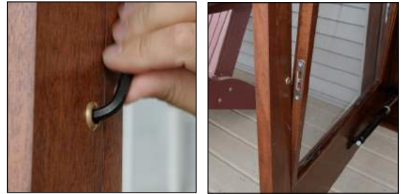
Screen/storm panel removal
