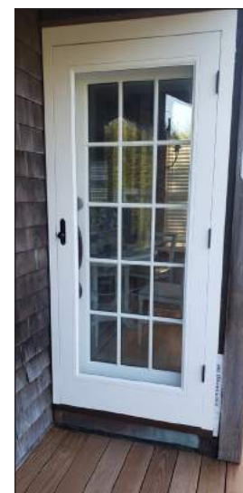
Drip kerf and beveled screen/storm to drain water off of the screen/storm door
